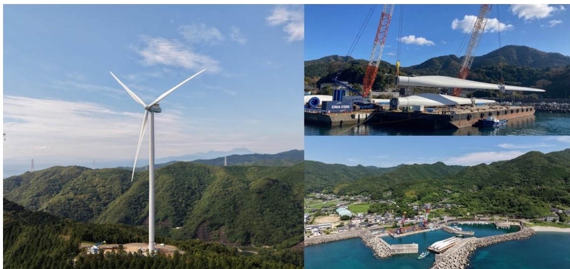
(Construction site and construction scenes of Reihoku Amakusa Wind Power Plant)
