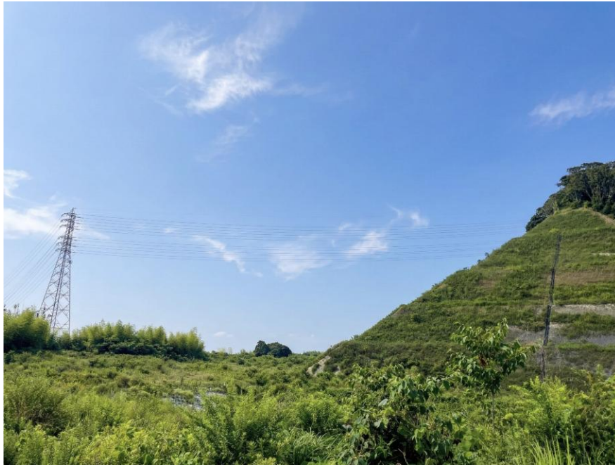
Planned Kikugawa Nishimura BESS construction site
