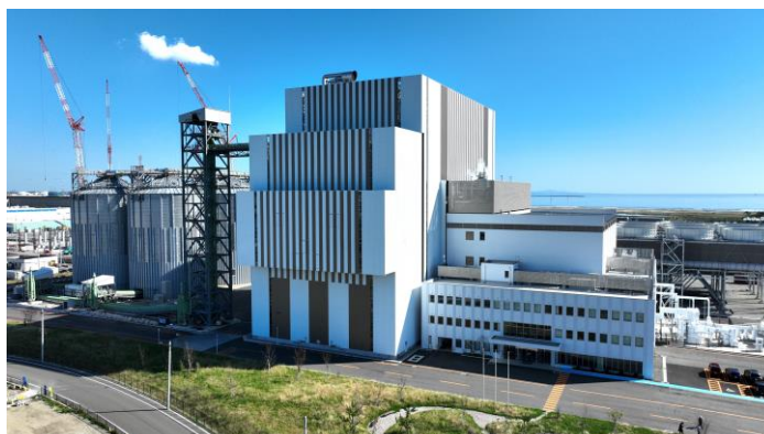
(Morinomiya Biomass Power Plant / Photo taken in October 2023)
