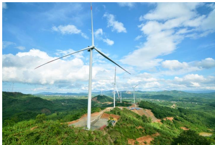
[Quang Tri Onshore Wind Power Project: Photo taken in July 2021]
